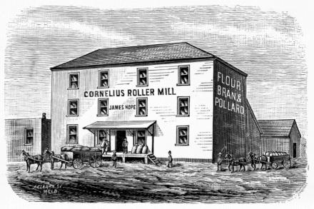
latest machinery, and on the most modern and best system which the progressive science of roller milling had been able to produce. In Mr. Hope's opinion this was indisputably the "Cornelius internal roller system." The new mill consists of a three-story building, 60 feet x 25 feet, with high, lofty floors, with skillion attached, 60 feet x 25 feet,
